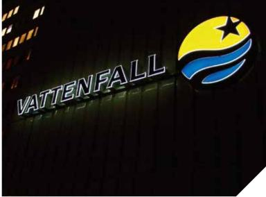
Channel letters with powder coated aluminum bottom. White interior with LED. 15 mm opal acrylic plastic front with or without vinyl top coating. Milled edges with 5 mm acrylic protrusion. Fronts screwed to letter sides. Power supply hidden inside the letter.
